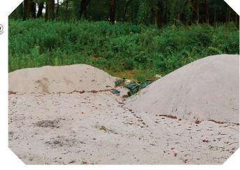
Piles of sand sitting on the ground and left uncovered can become contaminated with debris and are prope to loss.
